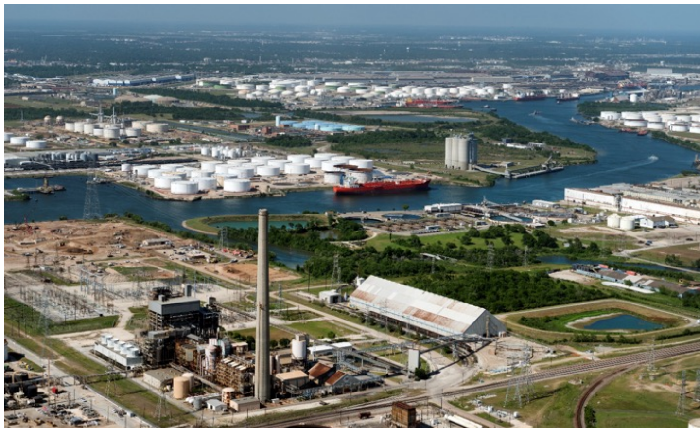
Aerial view in 2014 of the Houston Ship Channel and surrounding industrial areas in Houston, Texas. Credit: Carol M. Highsmith/CC BY-NC 2.0
